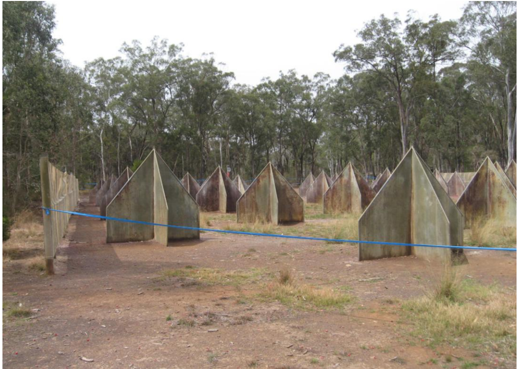
Figure 19 — a precinct in the paintball area featuring shields made from steel pipe and fibre-glass
