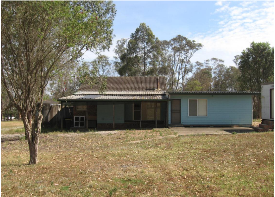
Figure 10 — south facade of the house at 68 Townson Road, showing rear and side extensions
