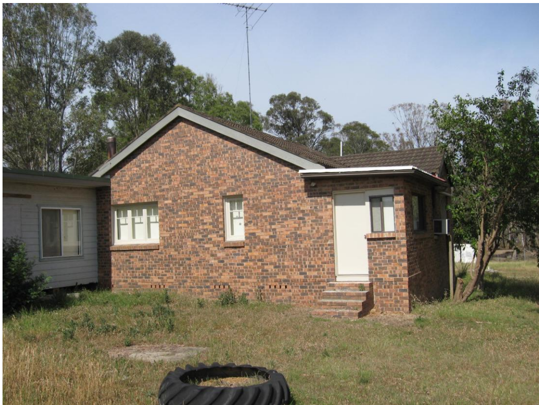
Figure 9 — east facade of the house at 68 Townson Road, showing the original form of the house, clad with newer bricks leaving the original windows.
